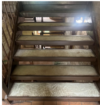
New stairs Building 2
